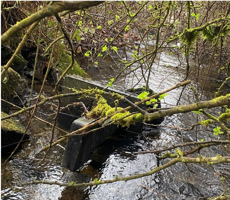
Figure 9.18: Representative photo of Grid Connection S3 - MANTUA_010, the 27 th of March 2025.
