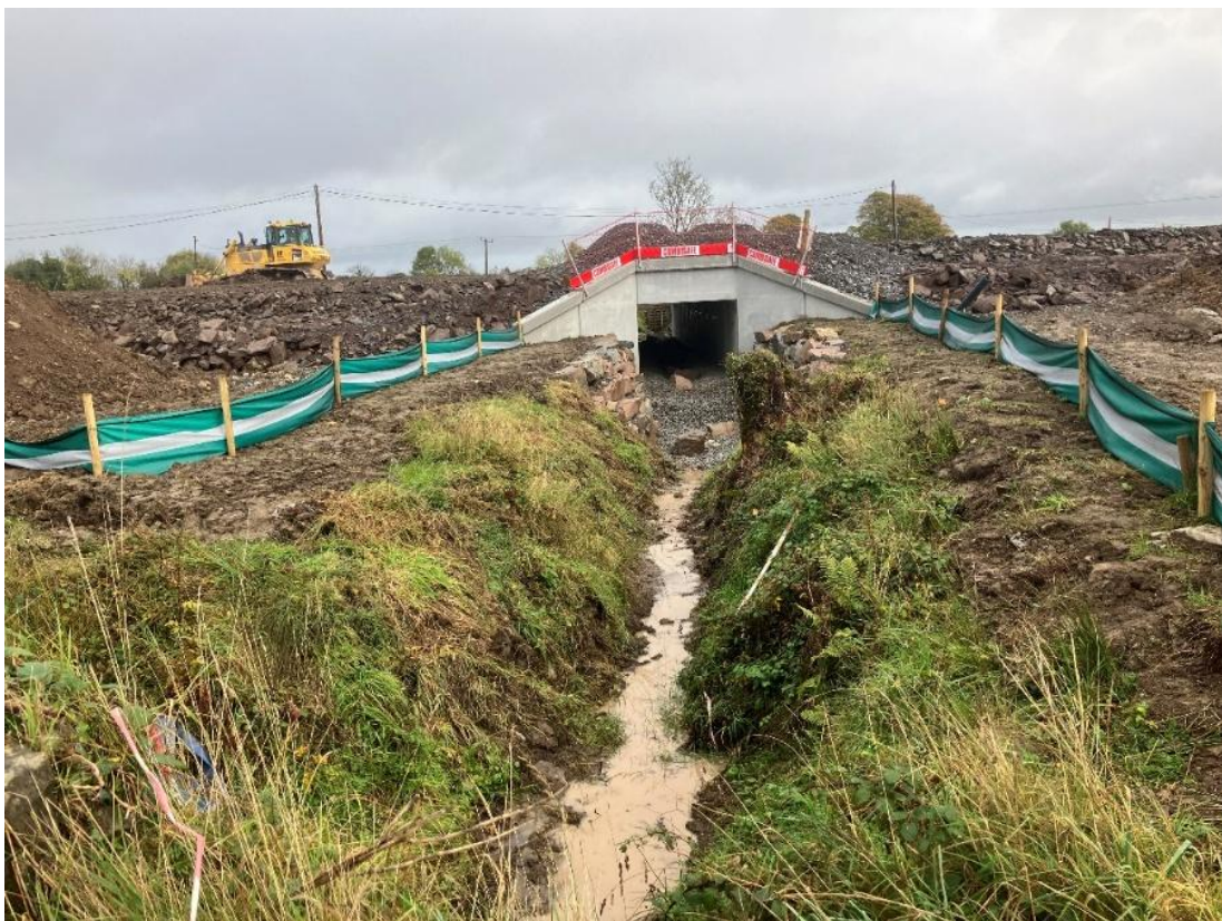
Figure 9.13: Representative photo of S13 - CARRICKNABRAHER_020 showing construction site, 17th of October 2024
